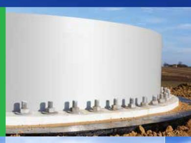
WIND TURBINE FOUNDATION. 20 sets of the versatile Tentec Aero WTF tensioners were used together with high pressure hoses and hydraulic tensioner pumps to have a productive rise of this wind turbine tower. In this case the wind tower base was held by two sets of bolts – M42 and M160.
